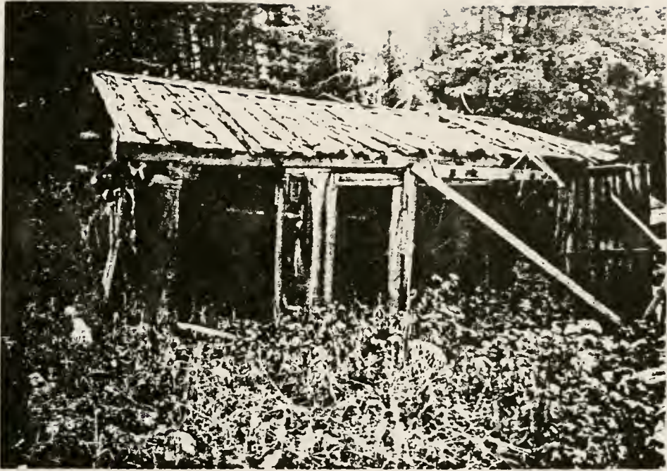
Figure 259. Stuart-Schultz Cabin (24PA410), east view of log-shed barn.
